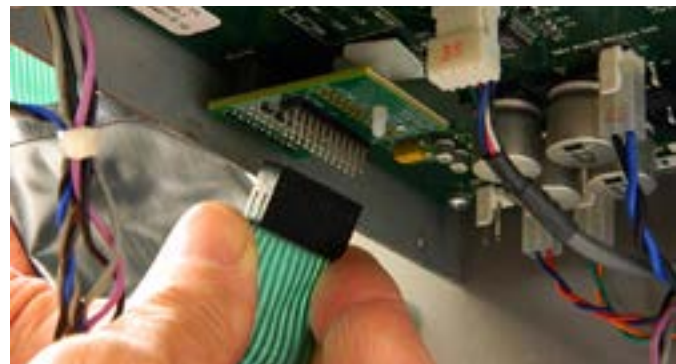
Step 15: Once the new EMI suppressor is attached, you can re-attach the green keypad cable.
