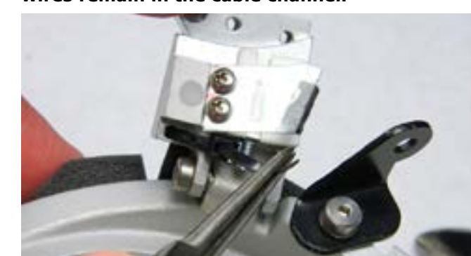
Step 20: With the needle nose pliers. You need to remove the tie wrap that you cut. This is slipped through 2 holes in the arm. This needs to be removed for the new cable tie wrap.
